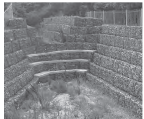
Using gabions to control water flow in a donga or gully
